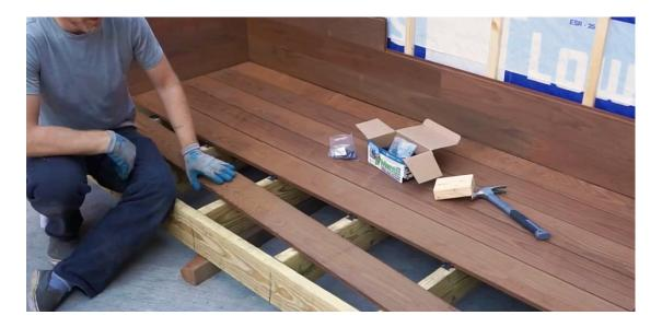
Minimum gap between boards: 3/16". Mantis®, TurboClip®, or Invisi-Fast® systems automatically space the boards. Clips must be matched to the groove that is milled.
